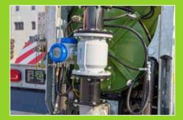
The flow rate during discharge is measured inductively by means of the Krohne Opti-flux 2300 digital flow meter.
